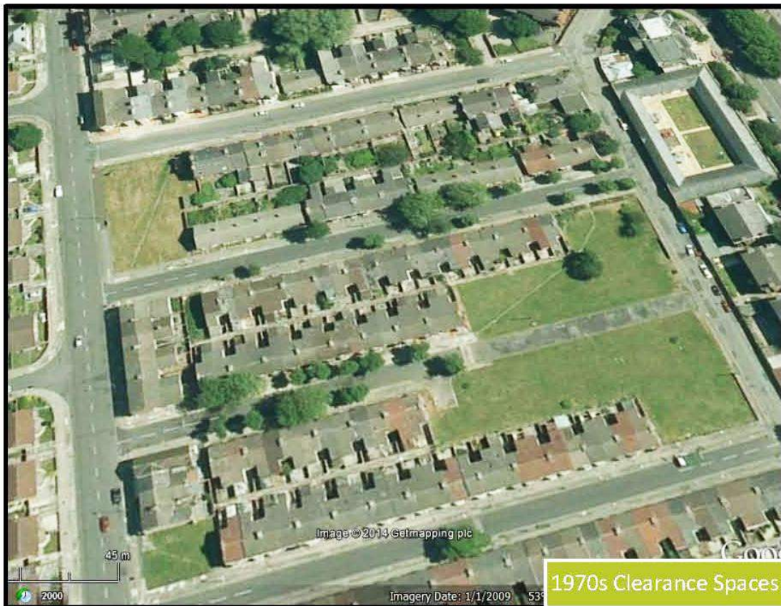
From Maisna Heritage Heritage Statement for SAVE, an aerial photograph showing the 1970s clearance sites within the Welsh Streets
